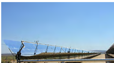
Figure 16.14 Parabolic trough collectors are used to generate electricity in southern California. (credit: kjkolb, Wikimedia Commons)
