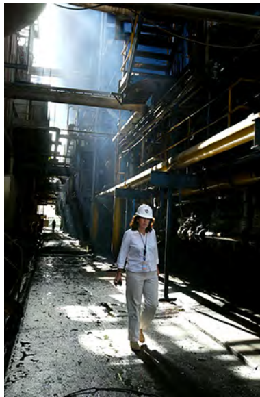
Figure 12.2 An engineer makes a site visit to the Baghdad South power plant.
