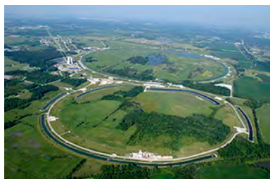
Figure 23.11 The Fermi National Accelerator Laboratory, near Batavia, Illinois, was a subatomic particle collider that accelerated protons and antiprotons to attain energies up to 1 Tev (a trillion electronvolts). The circular ponds near the rings were built to dissipate waste heat. This accelerator was shut down in September 2011. (credit: Fermilab, Reidar Hahn)
