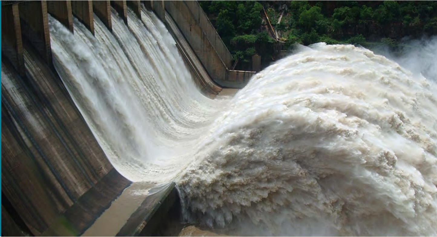
Figure 19.1 Electric energy in massive quantities is transmitted from this hydroelectric facility, the Srisaïlam power station located along the Krishna River in India, by the movement of charge—that is, by electric current. (credit: Chinto here, Wikimedia Commons)
